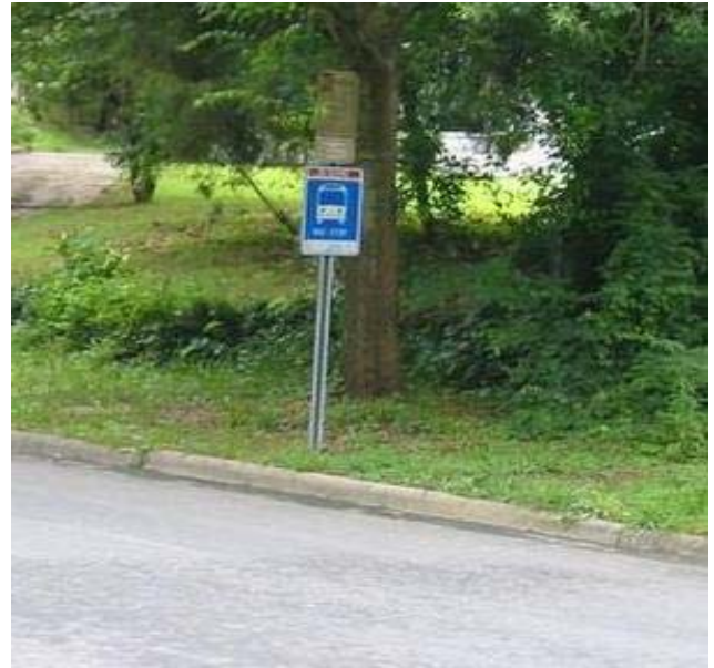
The picture above shows an example of a bus stop without a proper sidewalk, making access to the stop very difficult. A bench and proper shelter are also missing from this bus stop.
